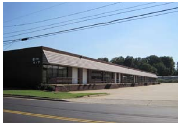
Renovated light industrial/flex space on Atando Avenue.
