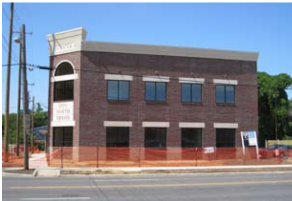
New office facility with good design characteristics under construction on North Tryon Street.
