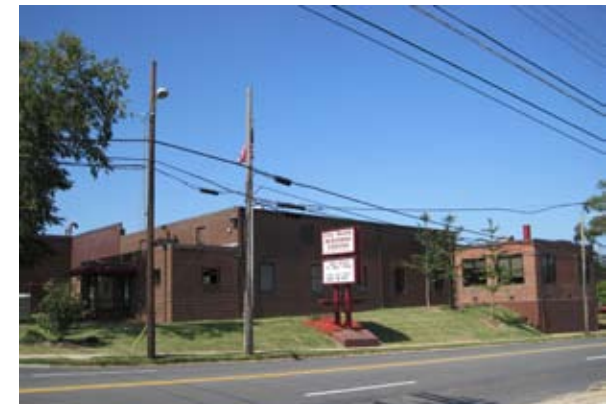
The City North Business Center has been redeveloped for a mix of retail, office, and light industrial uses.
