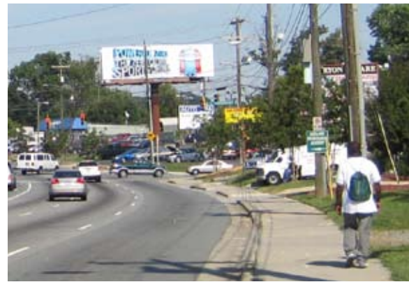
Sidewalks at the back of curb do not offer pedestrians safety from passing traffic.
