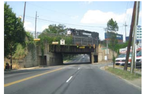
The 16th Street Railroad Bridge is a constraint to improved sidewalks, bike lanes, medians, and turn lanes.
