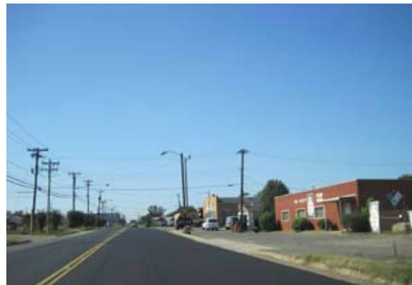
Atando Avenue has a number of continuing productive industrial, warehouse, and industrial uses.
