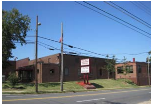
The City North Business Center has been redeveloped for a mix of retail, office, and light industrial uses.
