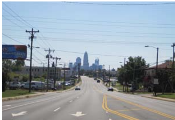
Portions of North Tryon Street have sufficient width for left turn lanes, although other amenities are lacking.
